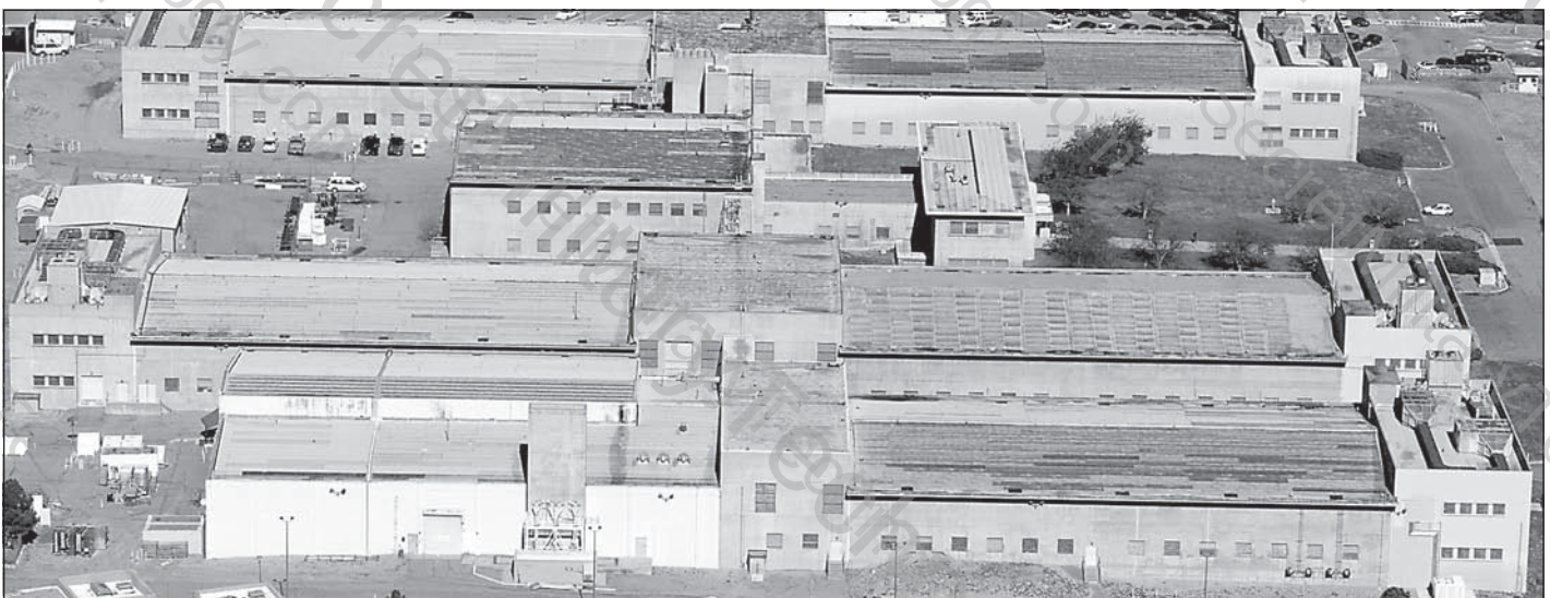
Figure 2: LANL's Chemistry and Metallurgy Research Facility
